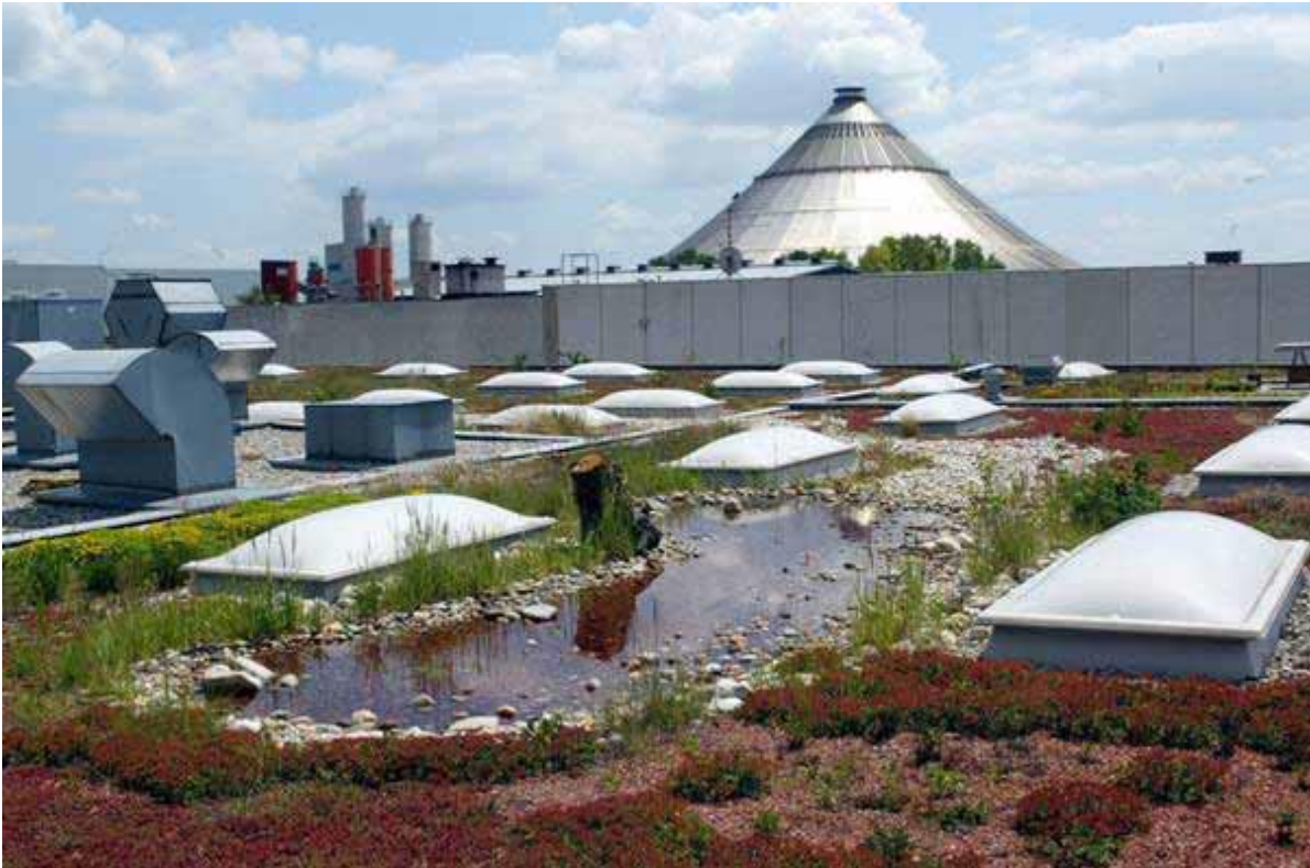
Figure 1: Extensive green roof with pond, source (© OPTIGRÜN)
