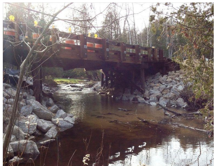
River after designing a proper crossing
