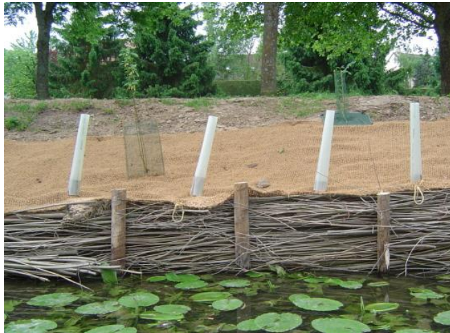
Example of natural bank stabilisation with wood weaving (France)
