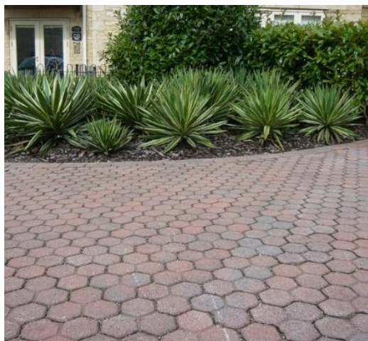
Example of permeable paving in Stamford, UK (photo courtesy of Susdrain)
